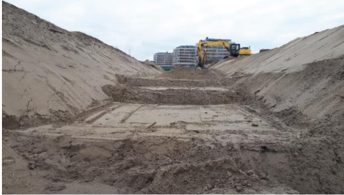
Verdichting fundering open bak
