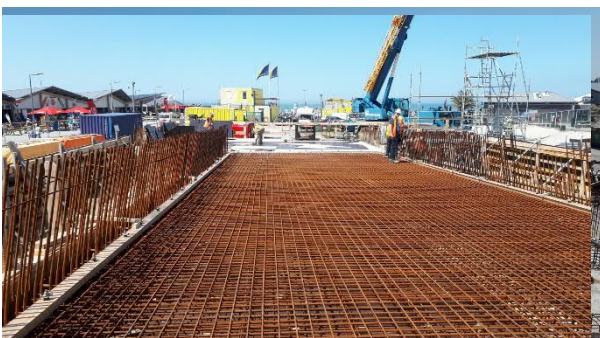
Bouw perrons station HvH Strand
